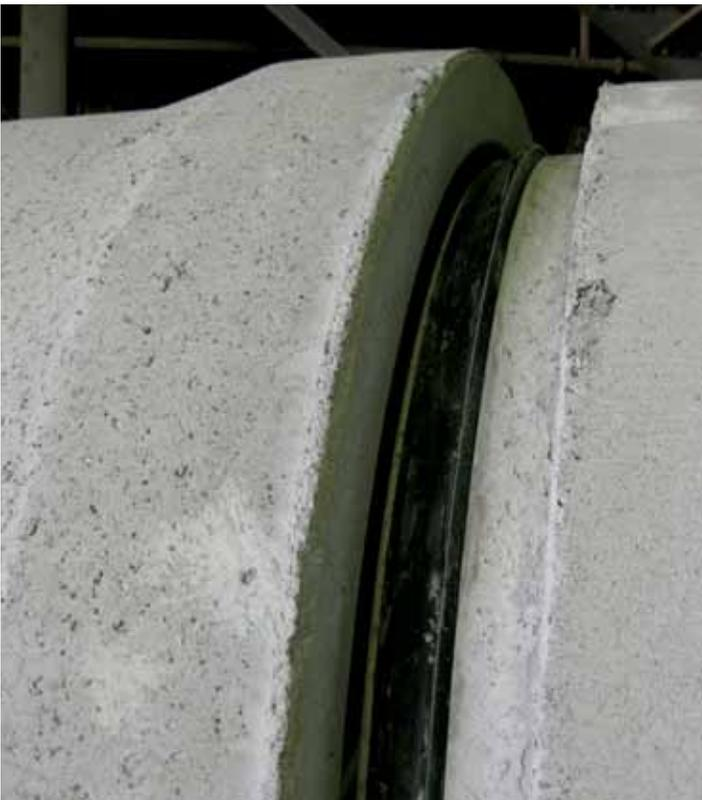
*Concrete pipe joint with rubber gasket*
