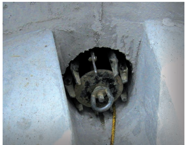
Mandrel test starting at a Maintenance Hole
